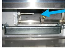
J-couple probe in exhaust duct collar as seen from below hood.
