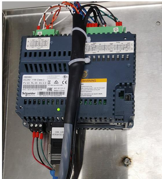
The Micro Processor is a programmable logic controller (PLC) located in the RPD-P-TC control panel. The sequence of operation, overrides, MAX AIR, and panel annunciation functions are all managed through the PLC. The integral HMI (Human Machine Interface) works as the command center for the TruFlow TC system.
