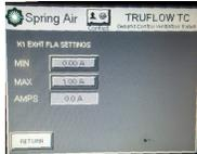
During the start-up of the exhaust fan, the minimum amps setting is to be determined by running VFD at minimum Hz. Record the actual **RUNNING AMPS** and enter the value recorded into the **MIN FLA**.
